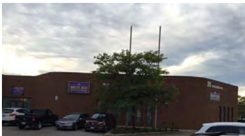
MOUNT ZION HOUSE OF PRAISE September 9/16 – Mount Zion House Of Praise, BRAMPTON, ON – 19 th Anniversary and Dedication of their new building – Pastor Richard Edwards
